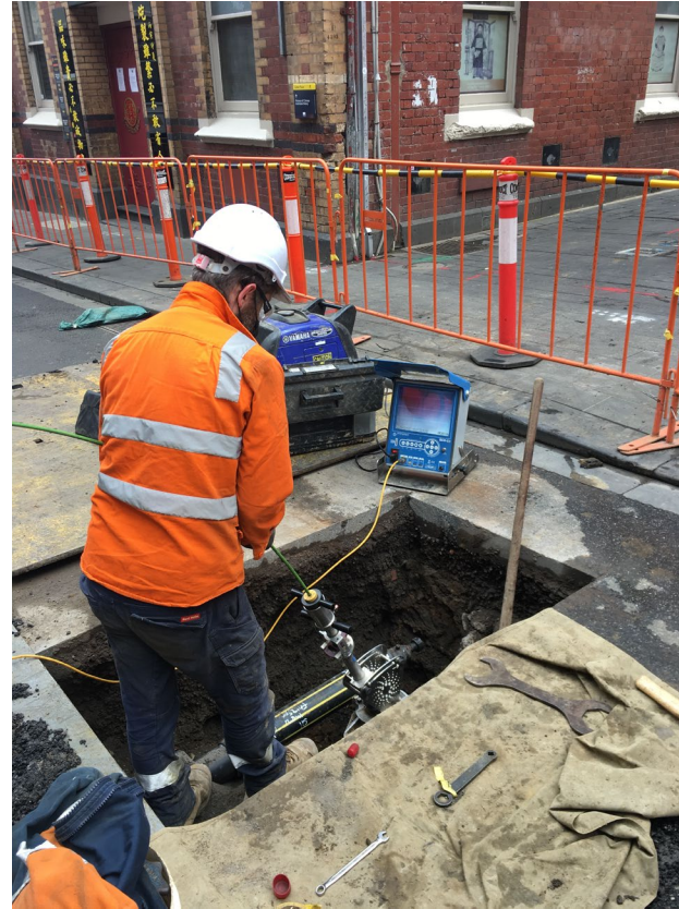
Inline camera inspection – Lt Bourke St (NE4) Diona
