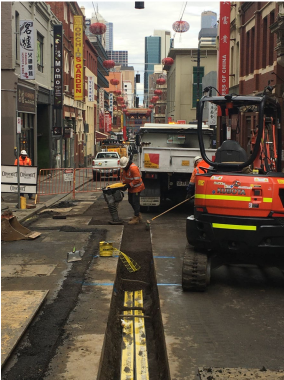
Compactions and Backfilling Open Cut Section Lt Bourke St
