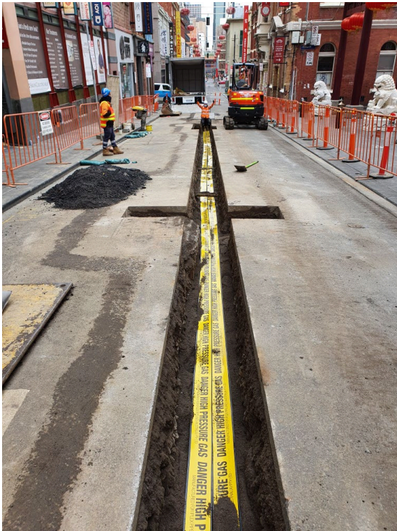
Installation of Warning Tape Open Cut Section Lt Bourke St
