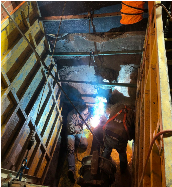
Welding of End Cap in Deep Excavation
