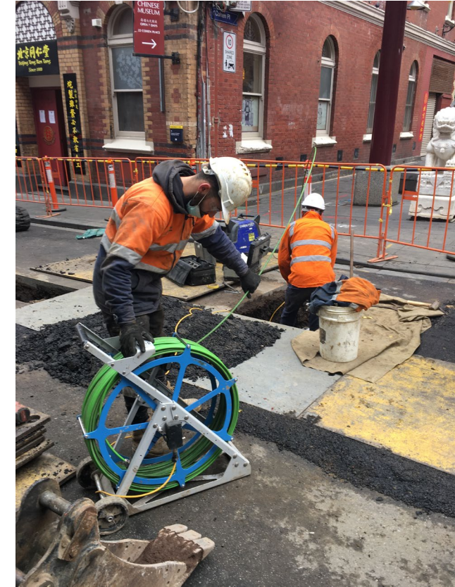
Inline camera inspection – Lt Bourke St (NE4) Diona
