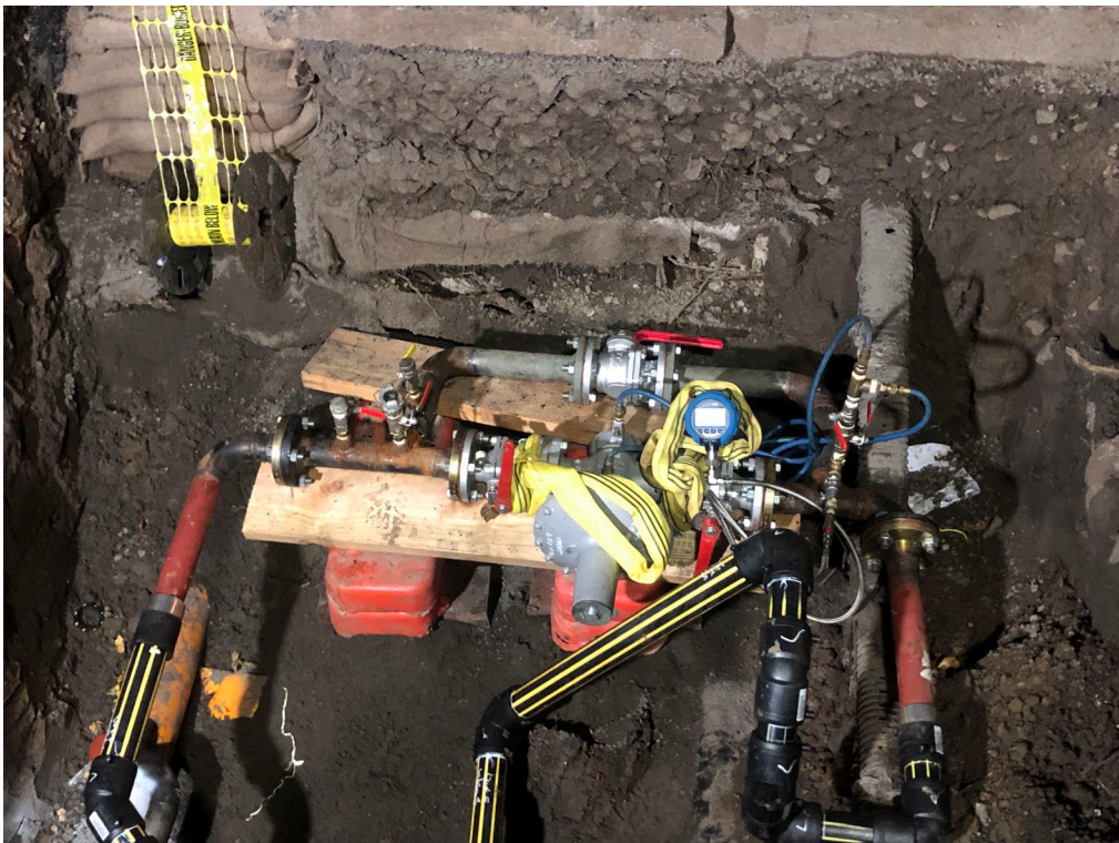
Temporary Regulator Setup Lt Collins St – Diona
