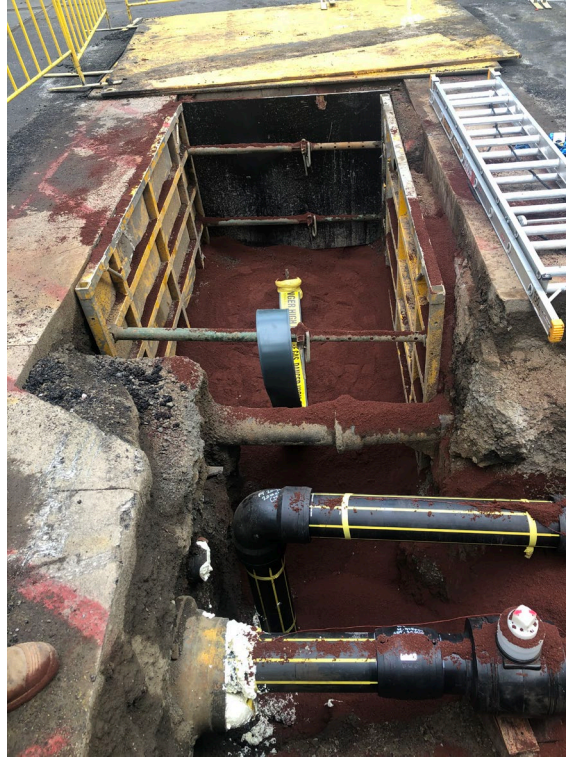
Road crossing with deep Excavation – using shoring plates for trench support
