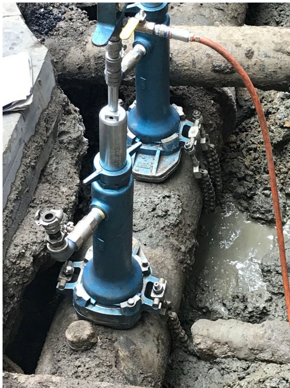
Wask Gears for Cut and Cap Preparing for Decommissioning
