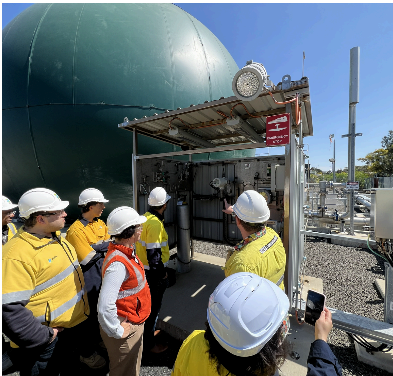
Malabar Biomethane Plant, source - Jemena
