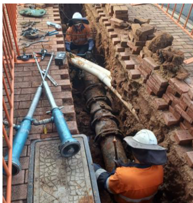
Pictured: Teams in the field working to upgrade legacy pipes.
