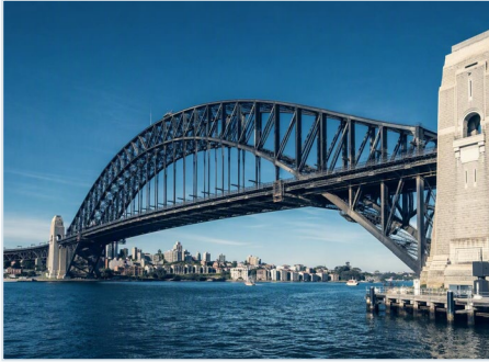
Sydney Harbour Bridge
