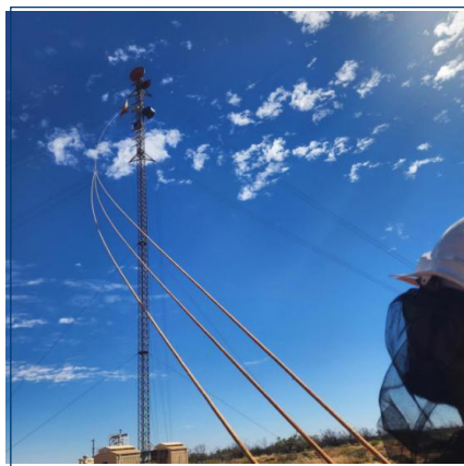
Field delivery of communications infrastructure renewal across remote DBP assets
