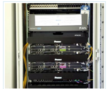
Communications infrastructure renewal
