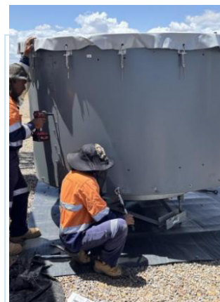
Field installation under live operating constraints
